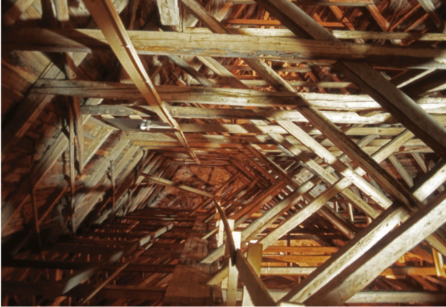
FIGURE 6 The roof structure of Pernaja church (1440d, 1452–1453d) PHOTO: LIVADY
